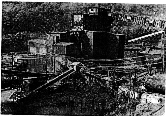
Top, Left: This is the most modern Anthracite Breaker still operating in Pennsylvania. It was built in the mid-1960s and still loads out about a hundred cars per day. Construction is steel framed with corrugated steel siding.
