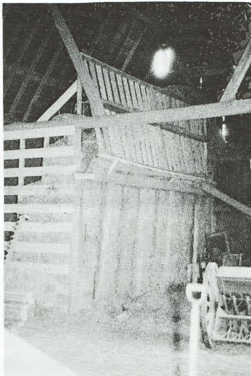
View of the straw mow retaining wall with the camera looking southeast. The actual original retaining wall, as drawn in the series, is found directly below the new upper portion you find on the right side of the straw mow. This is a picture of the area in which machinery is stored (see article). Photo: David Baxter.
