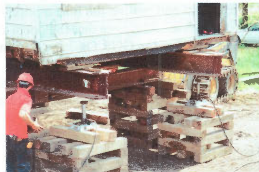
Above, preparing to move the north beam.
