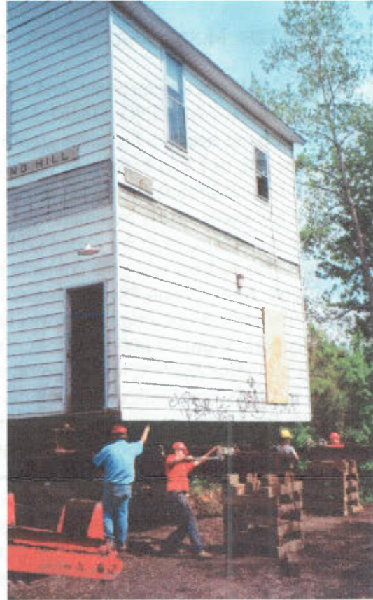
Next, the I beams were removed and the tower lowered using hydraulic jacks.
